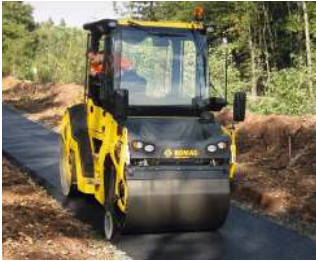
The BW 141 AD displays its compact operating capability in haul road construction.
