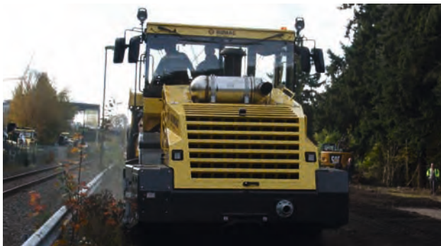
Work close to obstacles.
