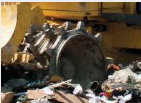
Scrapers guarantee clean wheels and high compaction.
