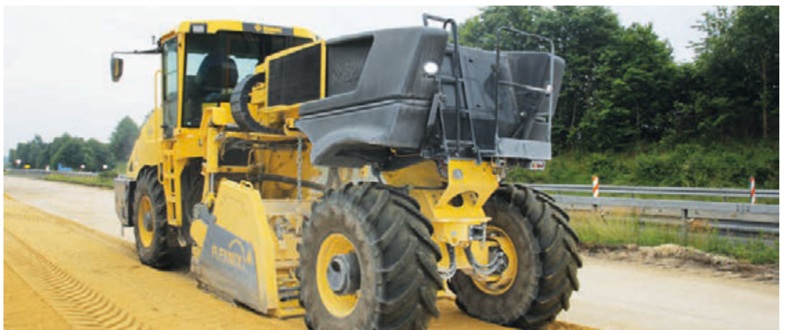
Milling a hydraulically bound base course.
