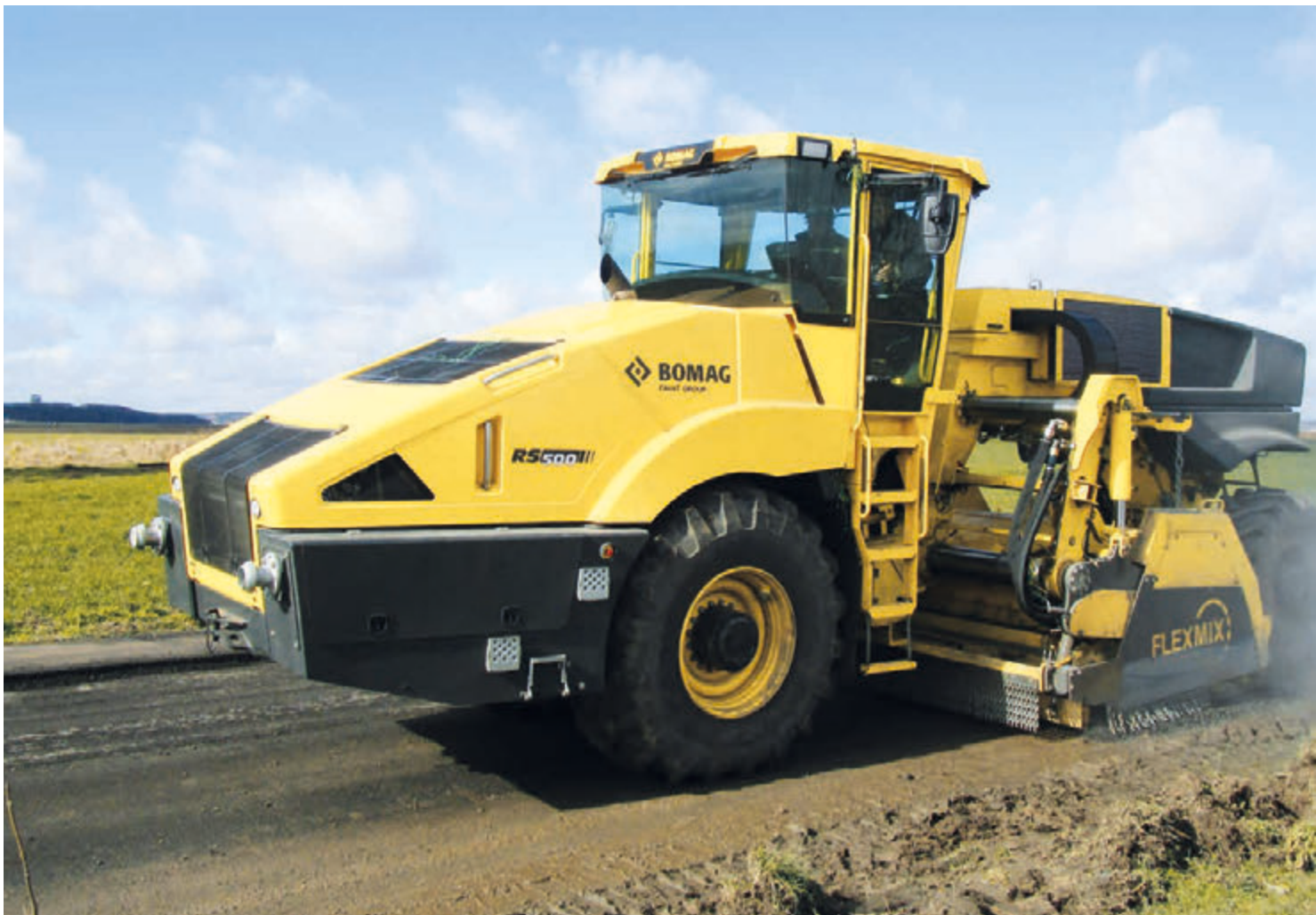
Milling 8 cm of asphalt road.
